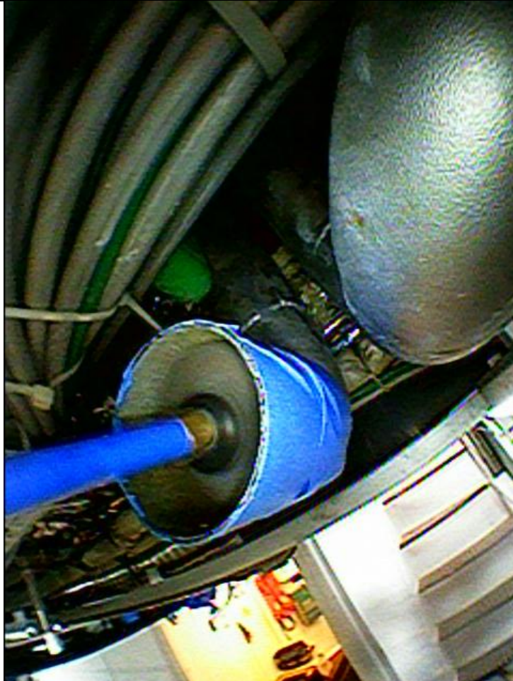
Mechanically cleaning the Pipe
