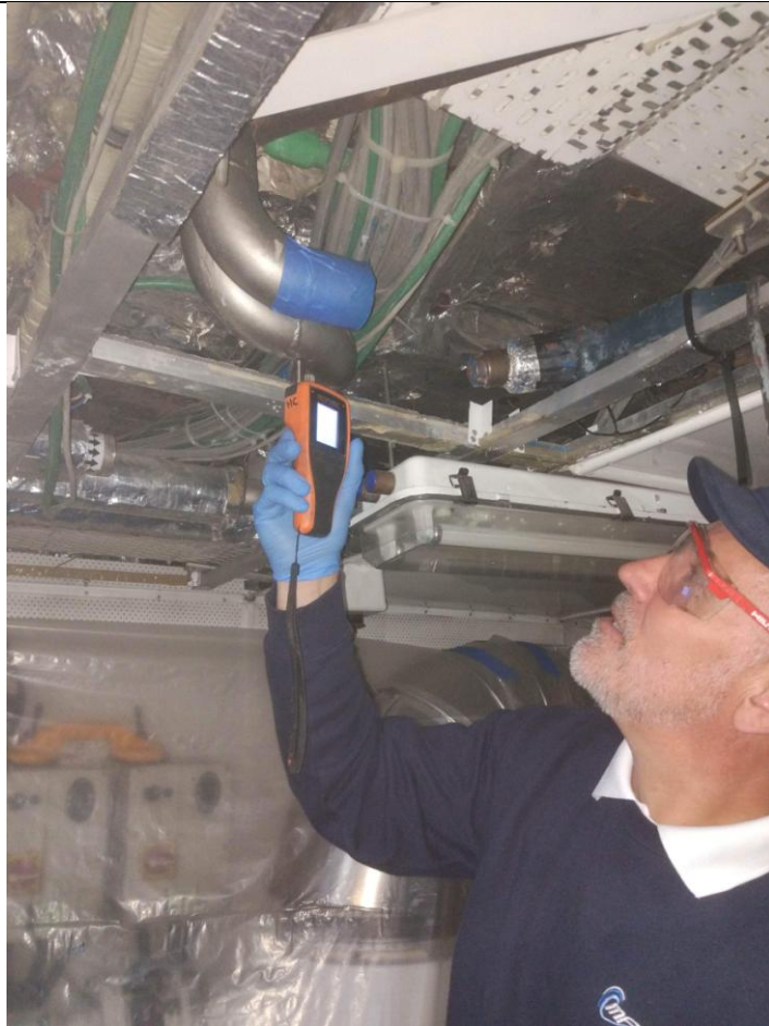
Pipe access was good in the ceiling of the engine room
