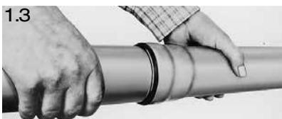
1.3 Centrally align socket and slip-in pipe and fit together by rotating slightly. Push in slip-in pipe until it meets socket ground.
