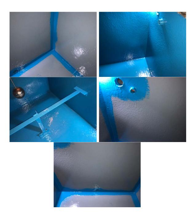
**TOP COAT** – The above was repeated with a top coat of ES 988 DWPU, again applied to all internal surfaces at a nominal thickness of 300-500 micron. As with the base coat, all critical seams were 'stripe' coated to build up the coating thickness in these areas.
