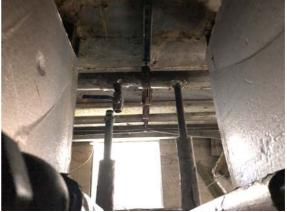
**ADDITIONAL WORKS** – The temporary tank and associated pipe work were drained and the pipework disconnected from the system as found at start of project.
