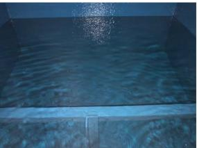
**DISINFECTION** – Once the coating had cured, the tank was refilled, disinfected with SuperSil and put back on line.
