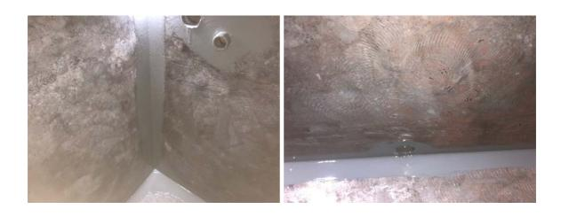
**BASE COAT** – The above was followed by an entire base coat of ES 988 DWPU, applied to all internal surfaces at a nominal thickness of 300-500 micron
