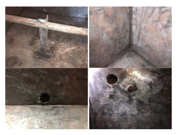
A stripe coat of ES 988 DWPU was then applied to all joints, seams and sharp edges to reinforce these critical areas and to allow the coating to be built up to 2-3mm.
